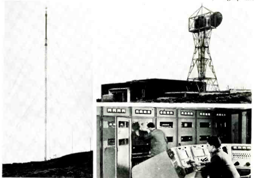
The BBC TV transmitter at Kirk o'Shott's, Scotland. Left: The 750-foot transmitting antenna. Upper right: TV programs relayed from London are received on these microwave parabolic antennas. Lower right: The 5-kw picture transmitter undergoing adjustments. The main operating console is in the foreground.
